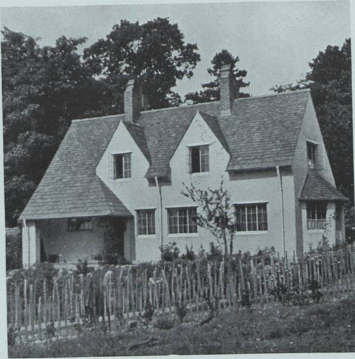
COTTAGE IN THE CLOSE, LLANFAIRFECHAN, N. WALES. ARCHITECT, H. L. NORTH, B.A., F.R.I.B.A., LLANFAIRFECHAN
