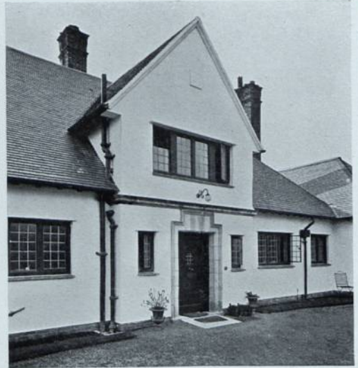
"THE BUNGALOW," CALDY, CHESHIRE—ENTRANCE FRONT. ARCHITECT, GILBERT FRASER, F.R.I.B.A., LIVERPOOL (Materials: Smooth cement face work; Storton stone to front door; leaded glazing and red tiles)
