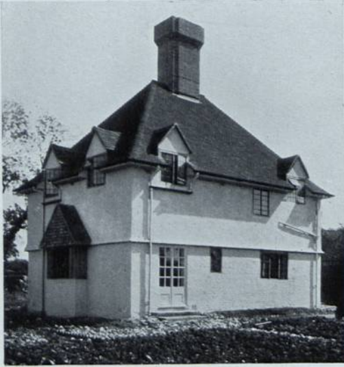
"HILL CREST," WILLINGDON, SUSSEX—REAR ELEVATION. ARCHITECT, JOHN D. CLARKE, F.R.I.B.A., EASTBOURNE (Materials: Walls brick, lower part dinged with lime, upper part rough plastered, the whole coloured warm cream; hand-made tiles on roof and hand-made bricks to chimney)
