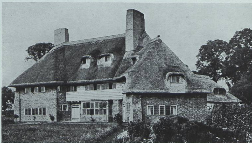
HOUSE IN WARWICKSHIRE. ARCHITECT, OLIVER HILL, F.R.I.B.A., 23, GOLDEN SQUARE, LONDON (see pages 53 and 54)
