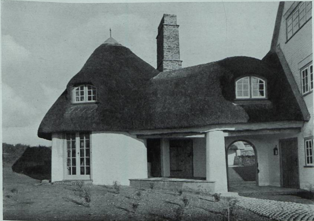
TWO ASPECTS OF A HOUSE AT CROYDE, N. DEVON. ARCHITECT, OLIVER HILL, F.R.I.B.A., 23, GOLDEN SQUARE, LONDON (see page 52) (Built on the coast in the traditional Devon farm-house style; whitewashed walls and reed thatched roof. Planned fan shape to form sheltered fore-court. Piers and chimneys in rubble stone; sitting room floor and doors in elm; first floor flooring in deal painted grey blue. Beams used in construction were recovered from a wreck.)
