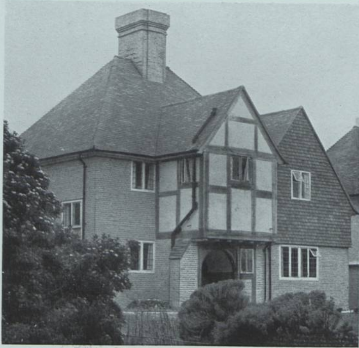
"OAK LODGE," WILLINGDON, SUSSEX. ARCHITECT, JOHN D. CLARKE, F.R.I.B.A., EASTBOURNE Materials: Silver grey hand-made 2-in. bricks, silver grey tile hanging, oak and plaster
