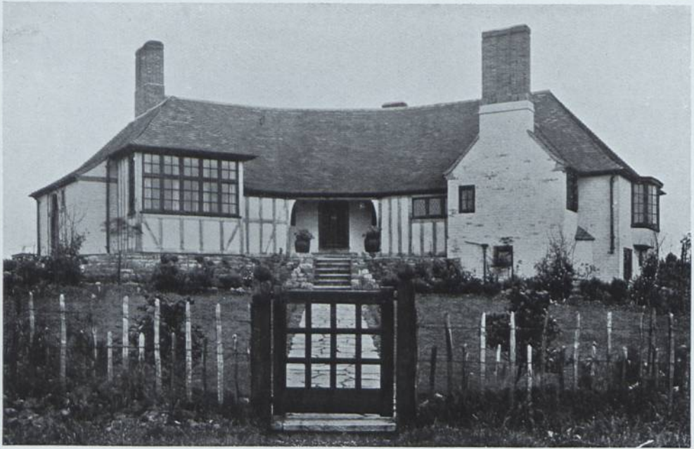
BUNGALOW AT BIRCHALL, LEEK. ARCHITECTS, R. T. LONGDEN, F.R.I.B.A., AND W. J. VENABLES, L.R.I.B.A., LEEK
