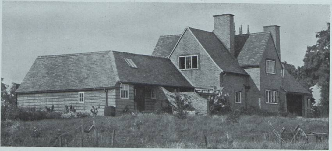
"MANOR COTTAGE," HAWTON, NOTTINGHAMSHIRE. ARCHITECT, A. P. STARKEY, HARROW. (see page 48)
