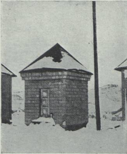
FIG. 7. Cell Concrete experimental House
