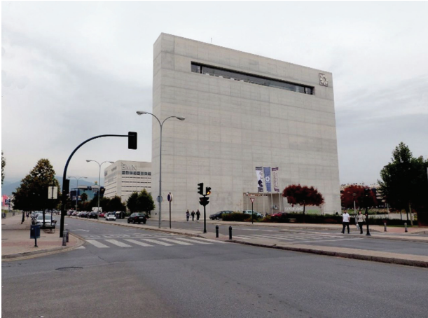
Fig. 3. Architectural complex (Cube & Museum, in the foreground) (photo by F.A. García Pérez, 2016)
