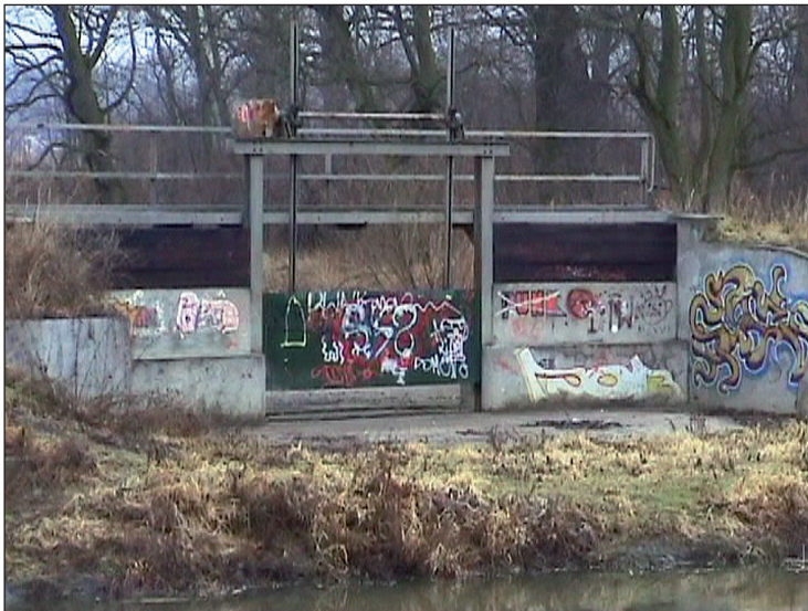
Fig. 4.15. Embankment sluice to Old Widawa (Photograph by S. Czaban)
