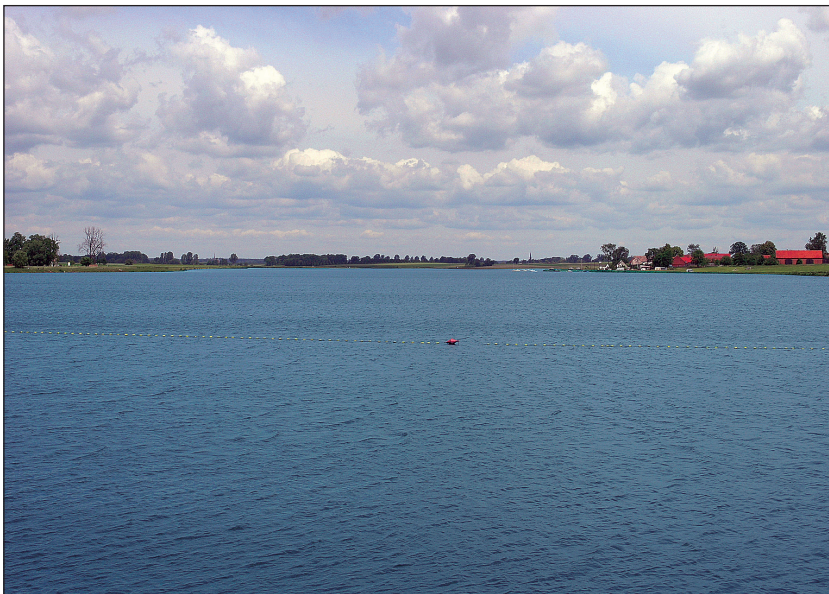
Fig. 4.16. View from the Michalice reservoir dam (Photograph by S. Czaban)
