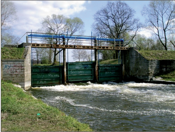
Fig. 4.14. Świniary gate –Widawa 6.618 km (Photograph by S. Czaban)
