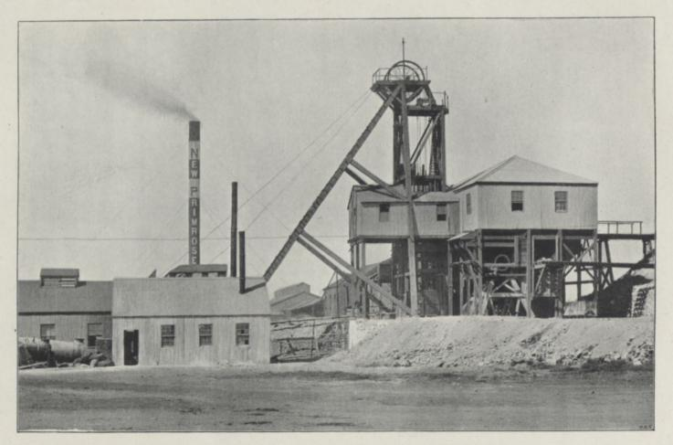
PLATE V.—HEADGEAR (VERTICAL SHAFT) AND SORTING-HOUSE, NEW PRIMROSE MINE.
