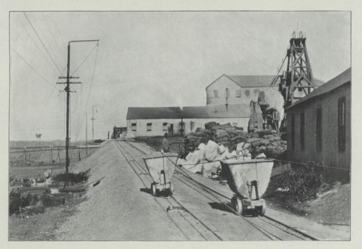
PLATE VIII.—TRANSPORT BY ENDLESS ROPE HAULAGE AT THE NEW PRIMROSE MINE.
