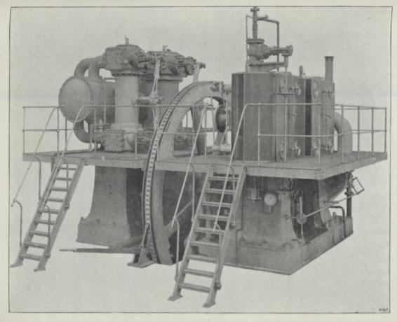
FIG. 63.—KING-RIEDLER AIR COMPRESSOR in use at the Robinson, Crown Deep, and Rose Deep. Steam pressure, 120 lbs.; air pressure, 80 lbs.; revolutions per minute, up to 90; capacity, 30 drills (No. 13 Slugger). King's patent engines fitted with Corliss valves and steam-jacketed. Riedler's patent air cylinders and valves; water-jacketed. Cut-off operated by combined speed and pressure governor.
