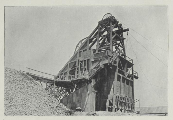
PLATE VII.—HEADGEAR (INCLINED SHAFT), ROBINSON MINE.
