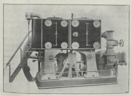
MILL ENGINE in use at the *Henry Nourse*. Compound-condensing—King type, Corliss valve gear. Steam cylinders, 19 in. and 30 in., diameter; stroke, 42 in.; revolutions per minute, 75; indicated horse-power, 330. Automatic cut-off in high-pressure cylinder to 70 per cent of the stroke. Hand cut-off in the low-pressure cylinder. Both cylinders steam-jacketed.
