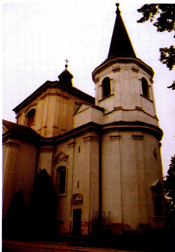
Fig. 6. View from the south-east
