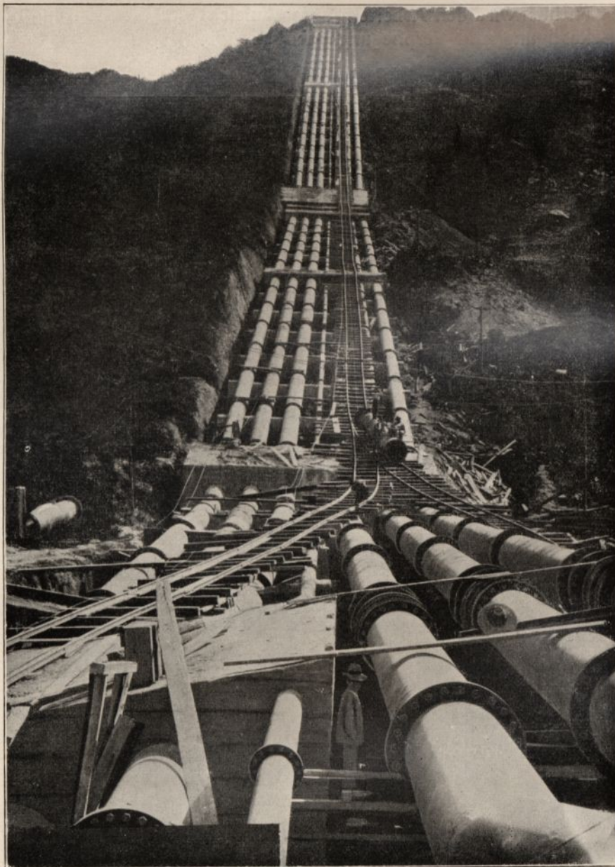
Druckrohranlage in Rio de Janeiro
