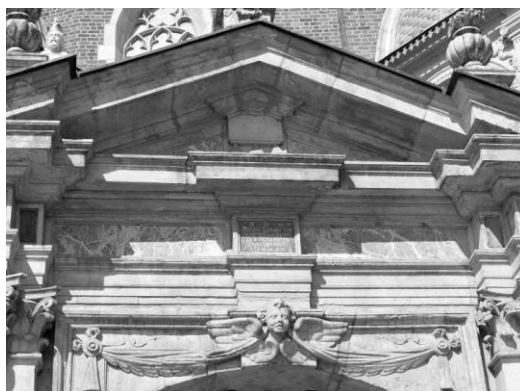
Fig. 11. Gate in the wall surrounding the Wawel Cathedral on the encrustations carried out Paczółtowiec “marble”
