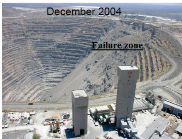
Fig. 4. Failure at Palabora mine (modified after Ngidi and Boshoff [18])
