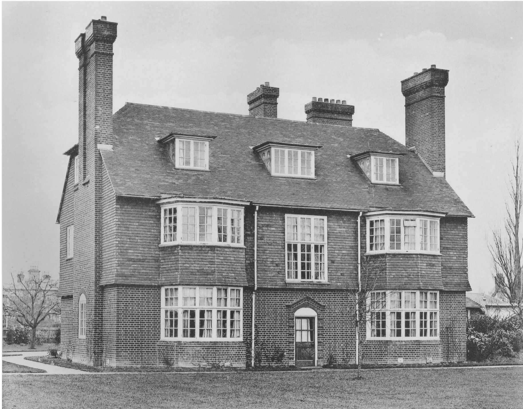
HOUSE No. I. GARDEN FRONT.
