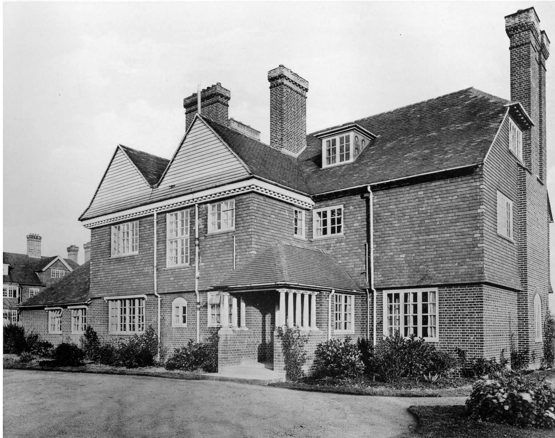
HOUSE No. I. ENTRANCE FRONT.
