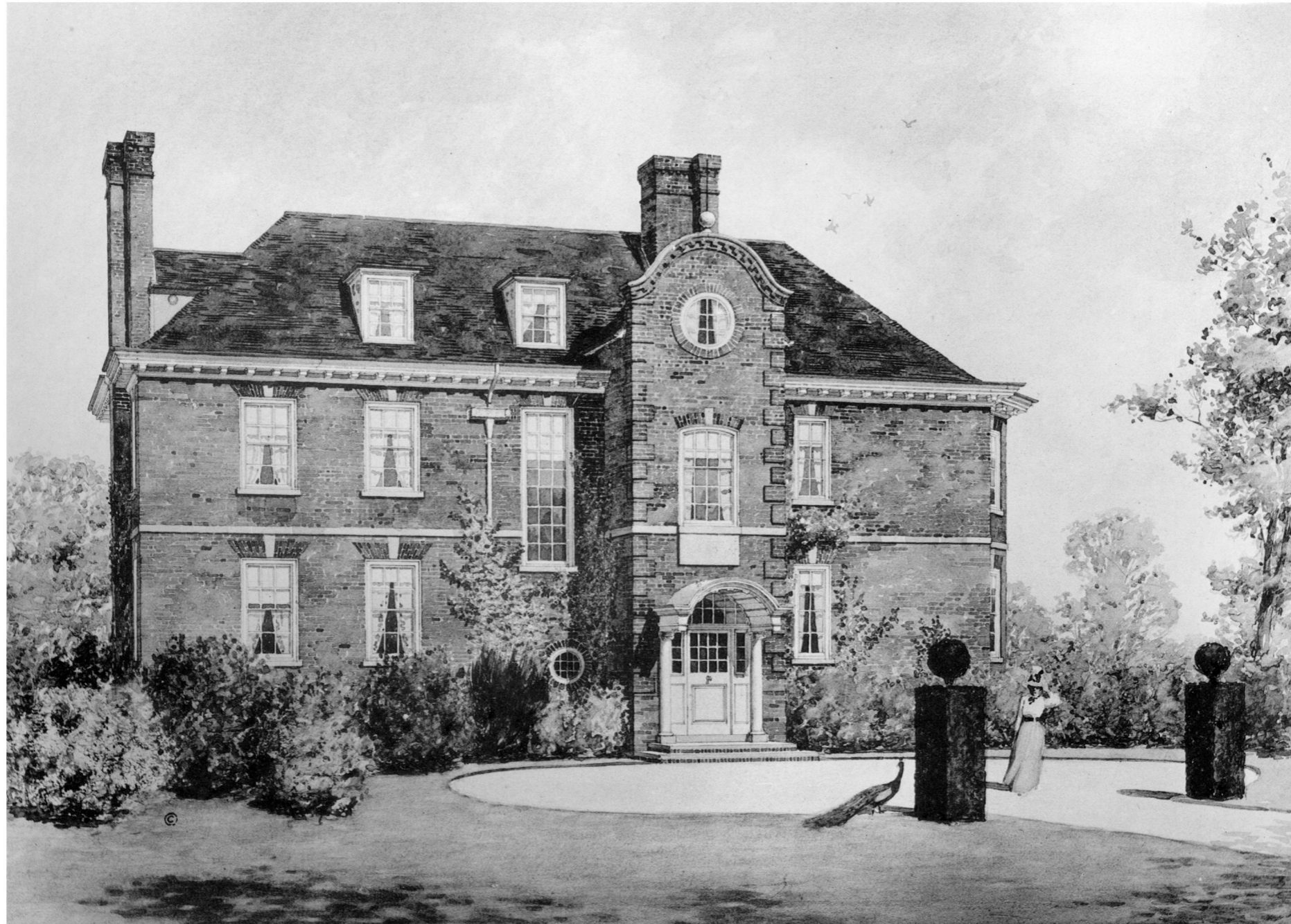
HOUSE No. XIX. ENTRANCE FRONT.
