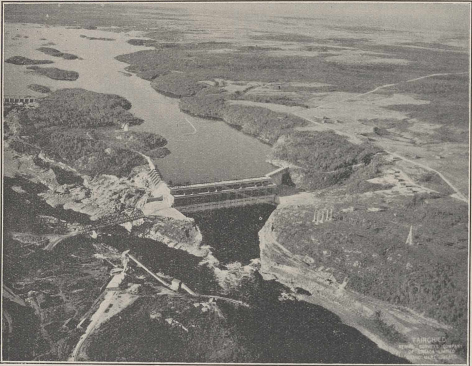
FIG. 1.—Hydro-electric installation (540,000 h.p.) at Isle Maligne, Lake St. John, Province of Quebec. (By courtesy of the High Commissioner of Canada.)
