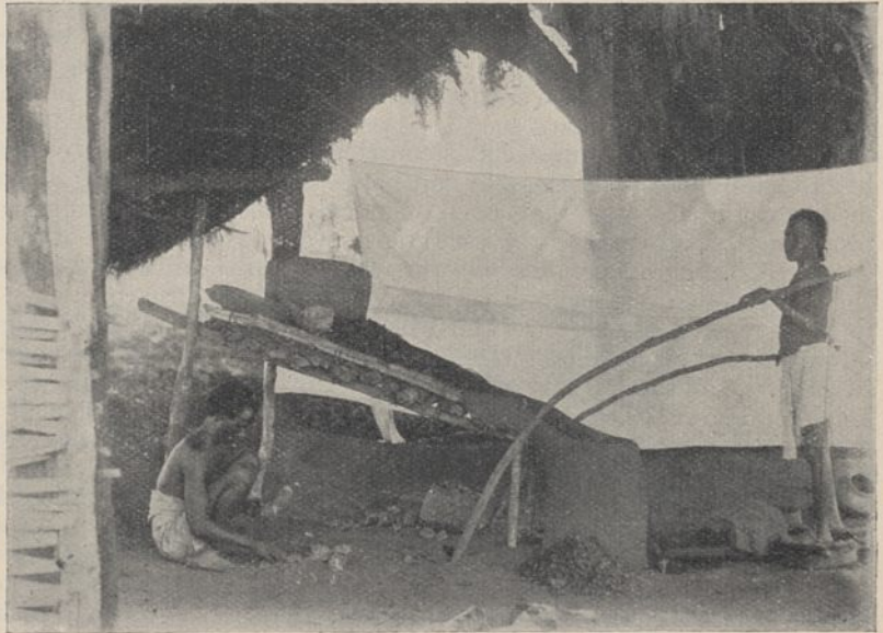
FIG. 3.—Bellows as used in India.
