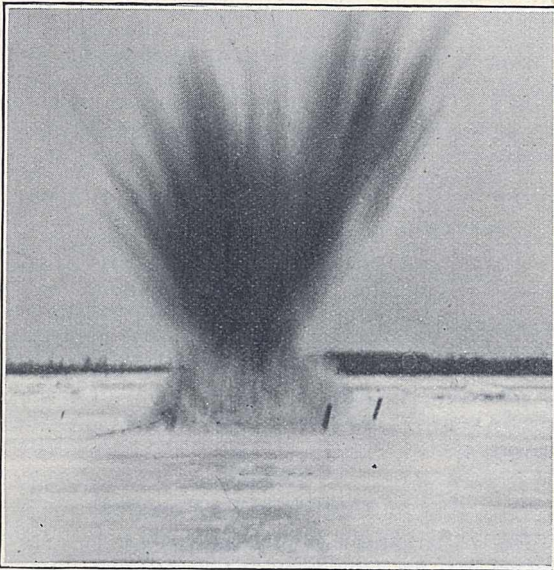
FIG. 1.—Ice exploding due to a charge of 90 lb. of thermit in the River St. Lawrence at Chimney Island, below Ogdensburg, N.Y. The mine was placed four feet down in slush-ice underhanging to a depth of eight feet the solid surface ice two feet thick. The bright flames forty-five feet high give a reversed image in the photograph, and, below, the disrupted ice is seen raised six feet. (Photo by W. A. Connolly, Morrisburg, Ontario.)
