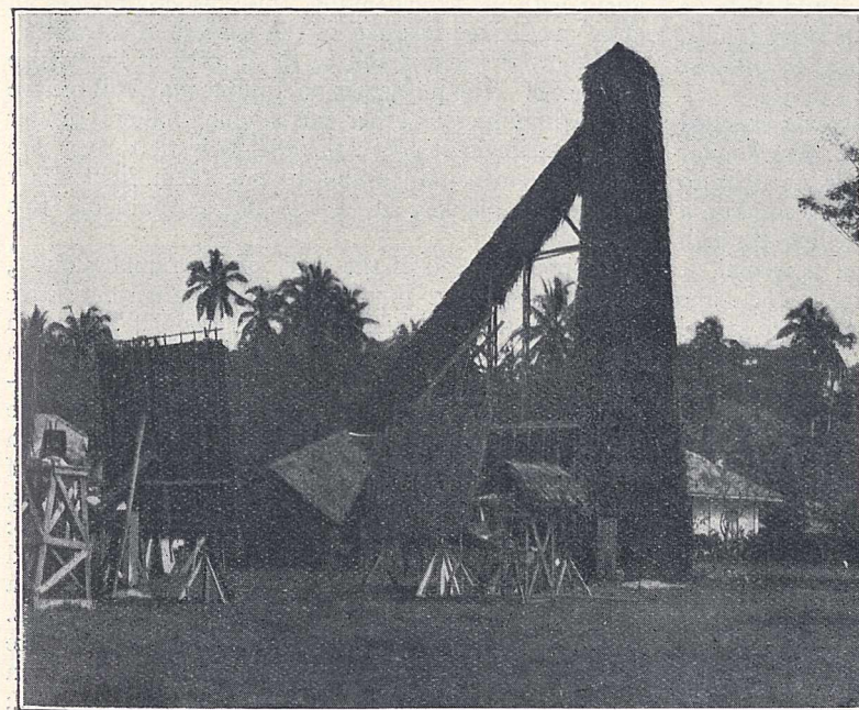
FIG. 4.—Prof. J. A. Miller's 63-foot tower telescope with the Einstein telescope in foreground.
