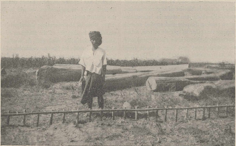
FIG. 2.—Bamboo stake fencing; usual type adopted since 1917. The stakes seen in picture originally stood 3 ft. out of the ground. From "Regulation of Rivers without Embankments."
