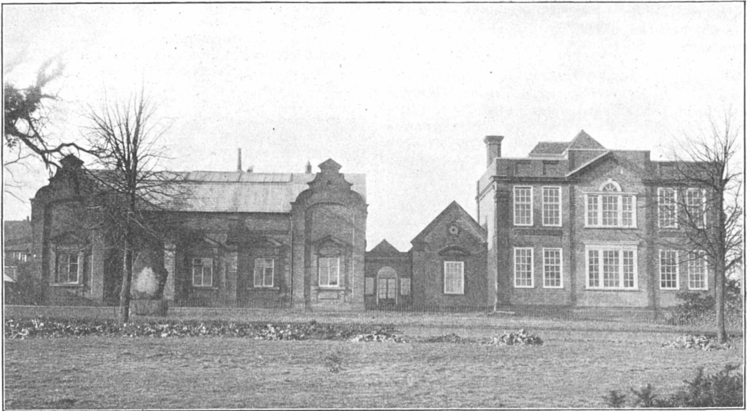
The new wing (on the right) adjoining the old one-storey building of the Rothamsted Experiment Station.
