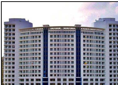
Photo 2. Newly developing district
