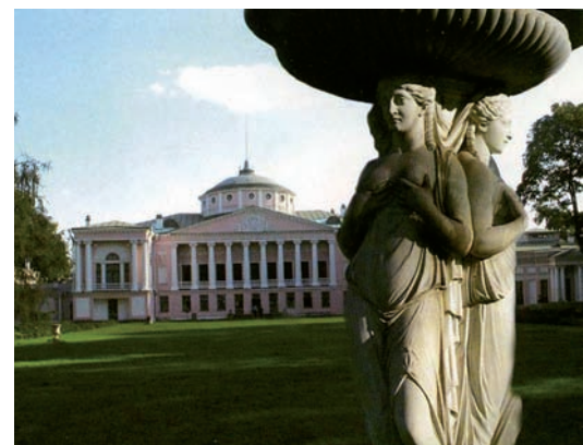
Fig. 5. Ostankino palace, the northern facade, the modern view
