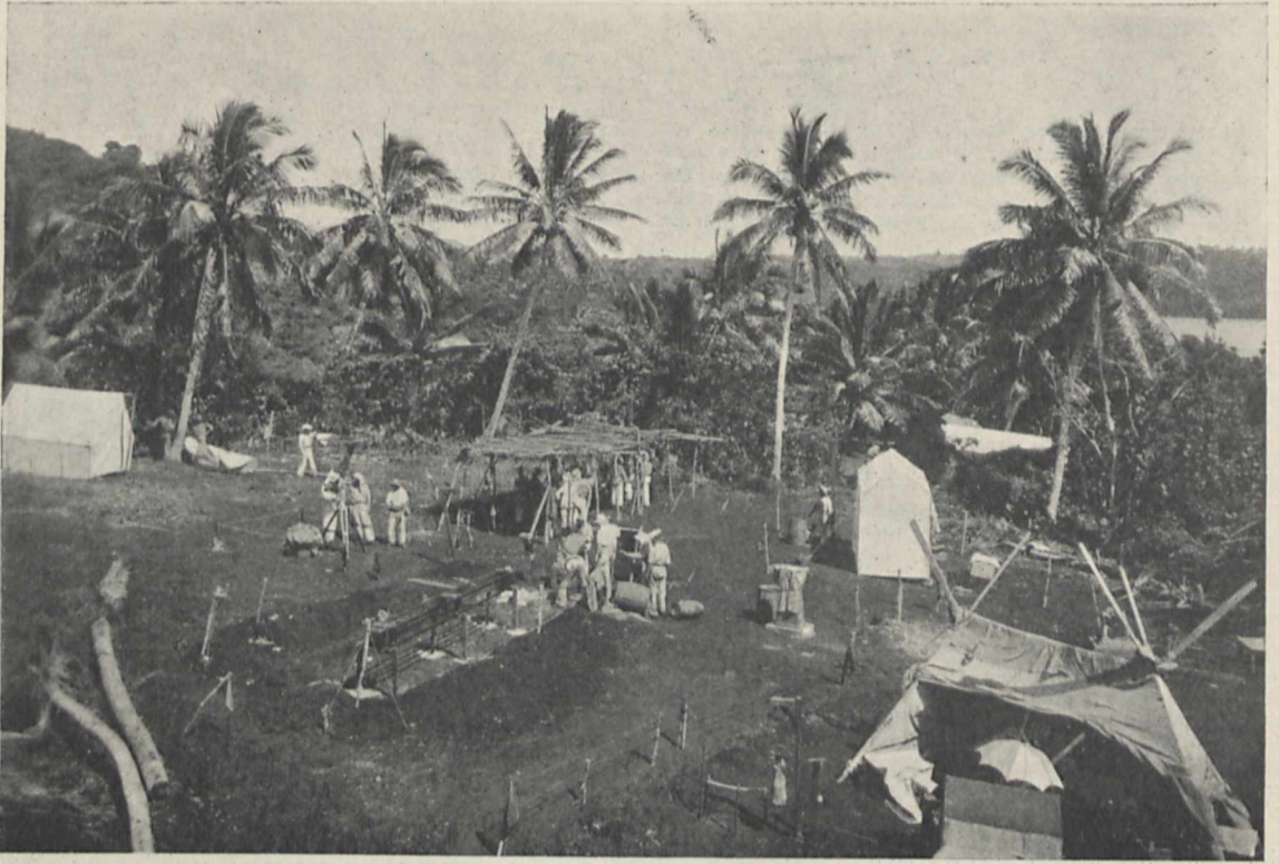
FIG. 2.—In the early stages of the erection of the Instruments. View taken from a Coconut Tree.
