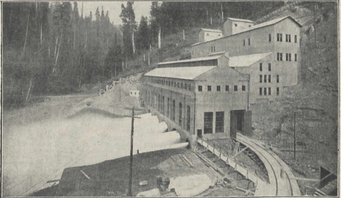
Hydro-electric Plant (developing 26,600 horse-power) on Puyallup River, near Electron, Washington.
