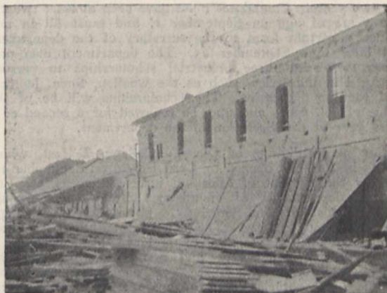
FIG. 1.—Railway station wall facing south.
