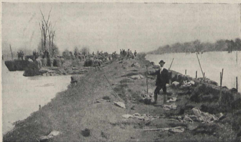
FIG. 2.—Repairing levee at Lagrange, Mississippi.
