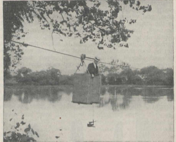
FIG. 2.—Cable and Car used to Measure Discharge of River.
