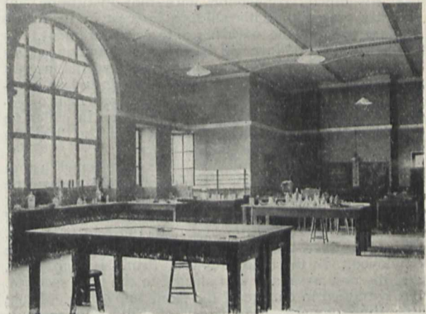
[FIG. 2.—Room No. 19 (General Laboratory).]
