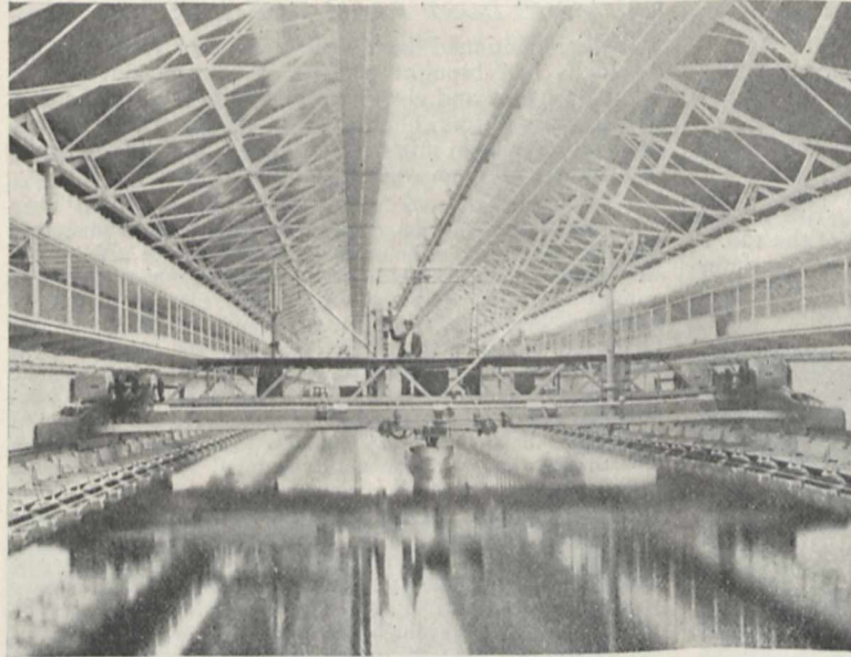
FIG. 2.—View of Carriage and Model at rest.
