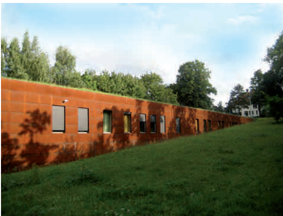
Fig. 1. RVU station group, MVRDV, Hilversum 1994–1997. Source: [7]
