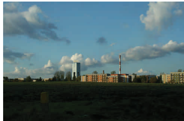
Fig. 11. Multi-family buildings in Bieruń Nowy with "Piast" mine shaft in the background (photo by I. Niedźwiecka-Filipiak, 2011)
