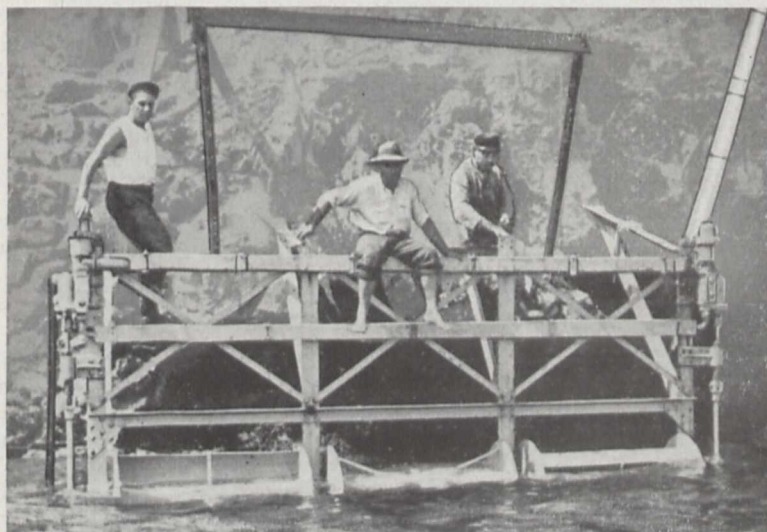
Fig. 2. Wellenrotor-Pumpanlage in Monaco
