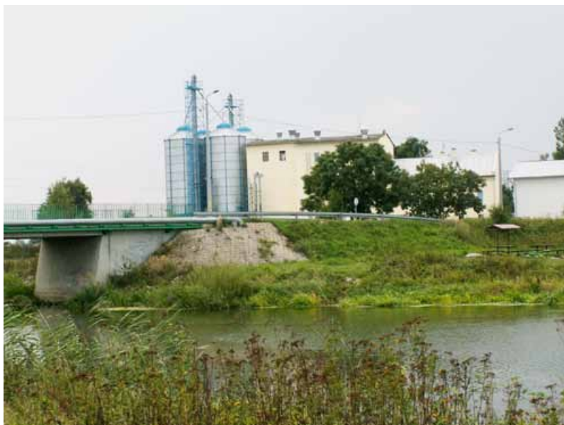
Fot. 124. Widok na zaadaptowany młyn od strony rzeki Oławy (fot. autorki) Photo 124. View of the adapted water mill from the River Oława (photo author)
