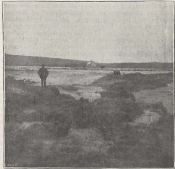
FIG. 2.—Broken roadway, with meadows submerged by the peat-flow, at Annagh Bridge. Foreground of heaped-up peat-mud and bog-timber. Lyne's cottage in the distance.
