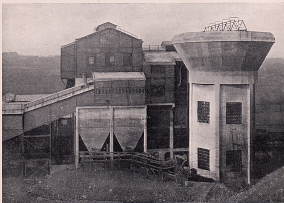
FIG. 8.—180 TONS PER HOUR WASHERY. NOTE THE LARGE CONCRETE SHALE BUNKERS WHICH RECEIVE DIRT FROM SCREEN AND WASHERY. A ROPEWAY CARRIES THE REFUSE FROM THERE TO TIP. ( Coppée Co. (Gt. Britain), Ltd. )
