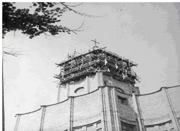
Fig. 6 Building of the reinforced concrete tower top [1]
