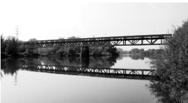
Fig. 4. The railway bridge over the Oder between Krapkowice and Otmęt. The western span fell down during the July 1997 flood. It was repaired but the traffic has not been restored (photo: M. Konopka, 2009)
