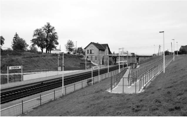
Fig. 10. Łosiów station on the Opole – Wrocław line, rebuilt in 2005–2006 as a passenger stop. Platforms were rebuilt, monumental wheelchair ramps were built, the loading ramp and additional tracks were removed. The building was left unchanged (photo: M. Konopka, 2009)
