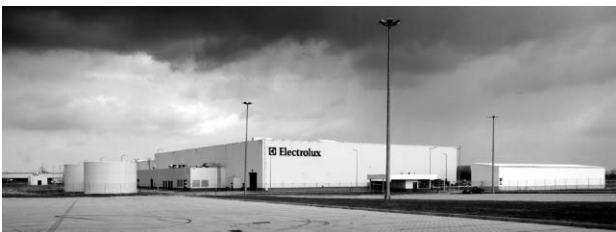
Fig. 2. Electrolux in Świdnica. View from the main employees parking towards the factory entrance (photo: M. Baborska-Narożny)
