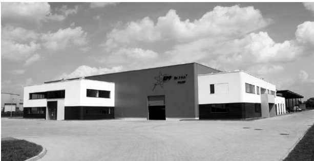
Fig. 15. EPP in Jelcz Laskowice. Production hall with adjacent separate functional parts: administration and social (photo M. Baborska-Narożny)
