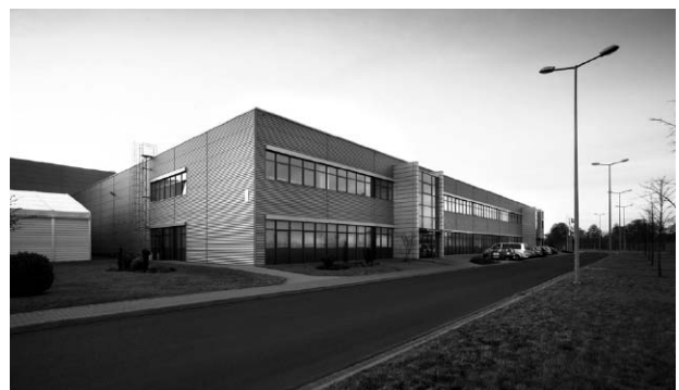
Fig. 4. Bosch in Mirków. Entrance building with social and administration functions (photo M. Baborska-Narożny)
