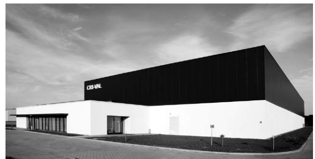
Fig. 13. Cri-val in Jelcz Laskowice. A smooth blend of administration-social building with production hall (photo M. Baborska-Narożny)
