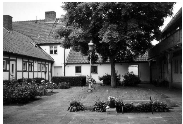
Fig. 8. Residential complex with the nest arrangement in Ystad, Sweden (photo: E. Cisek)
