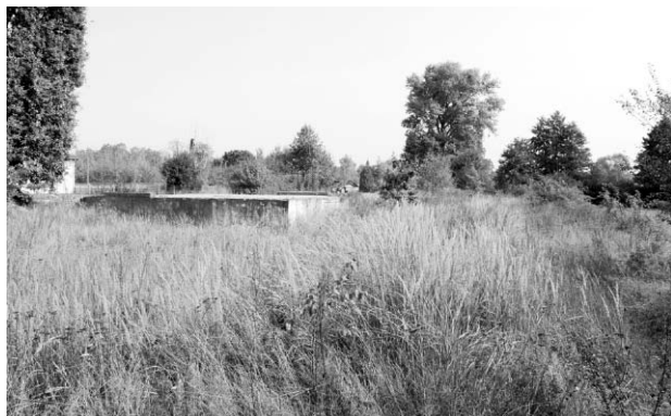
Fig. 6. Zielina station. The station buildings have been torn down. Only fragments of the ramp have remained (photo: M. Konopka, 2009)
