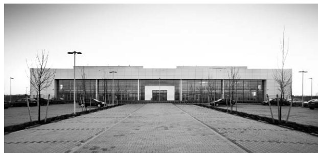
Fig. 17. Eto-magnetic in Wrocław. The entrance facade (photo M. Baborska-Narożny)
