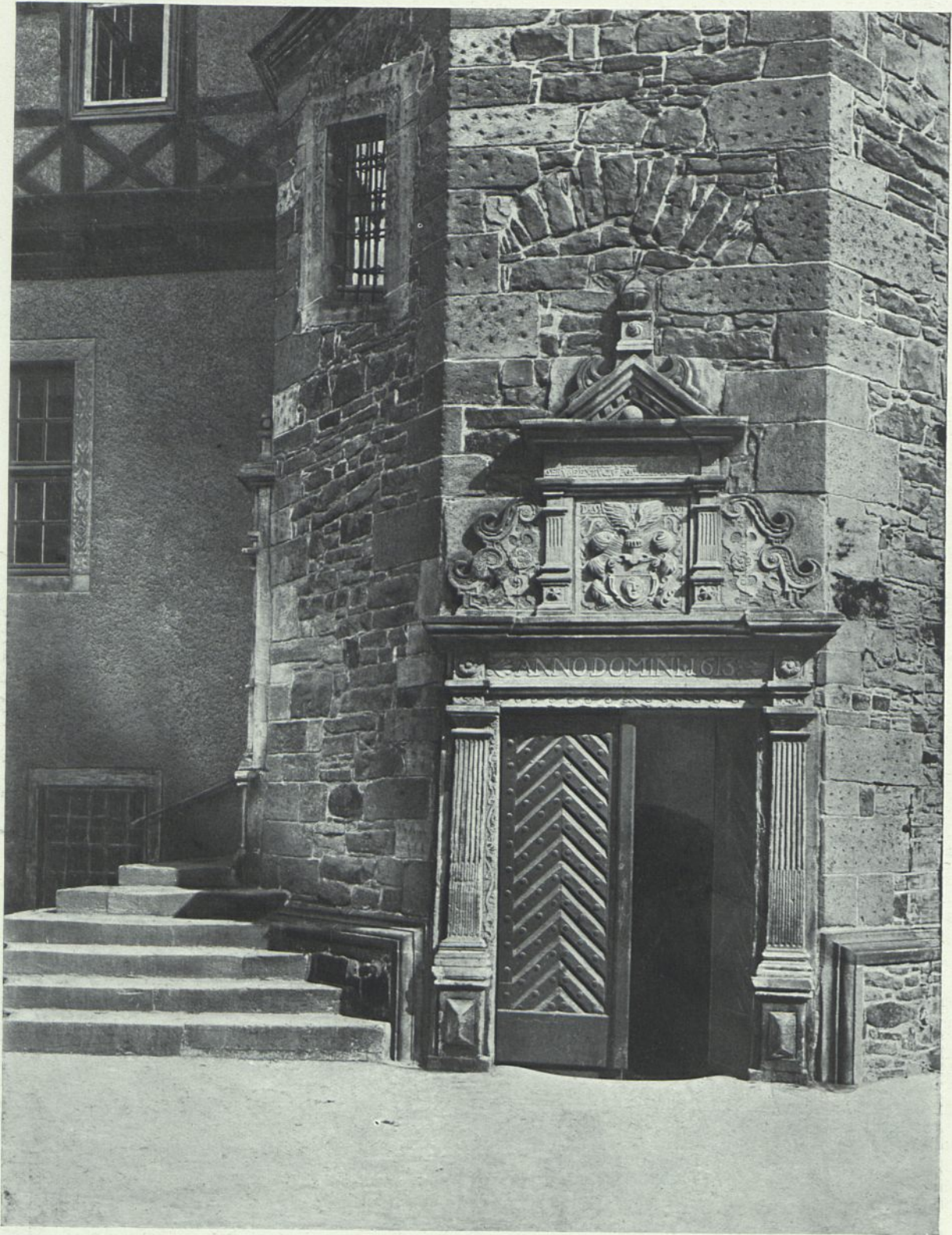
16. Rathaus in Höxter. Tür am Treppenturm.
