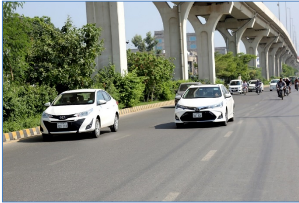
Fig. 7. A view of Bosan Road
