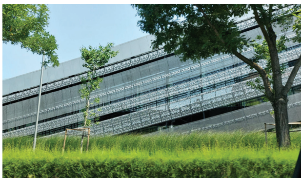
Fig. 9. Budapest, Ethnographic Museum – detail of the metal lattice on the glass exterior wall (photo by M. Wdowiarz-Bilska)
