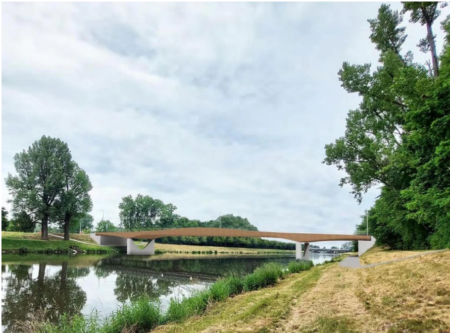
Fig. 6. New look of Kapitán Bartoš bridge [12]
