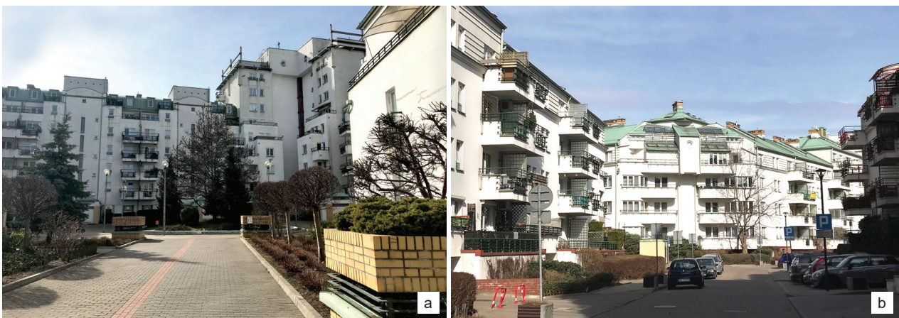
Fig. 5. The residential development at the National Education Commission Avenue 98 in Warsaw – an example of the realization of the postmodernism assumptions, characterized by a return to the quarter development with individualized, loosely interpreted, historical detail: a) view of the inner courtyard with interestingly arranged green zones and elements of small architecture, b) view of the development from the Artystów Street showing the gradation of the height of the development and illustrating the formal and spatial solutions used (photo by M. Wiśniewska)
