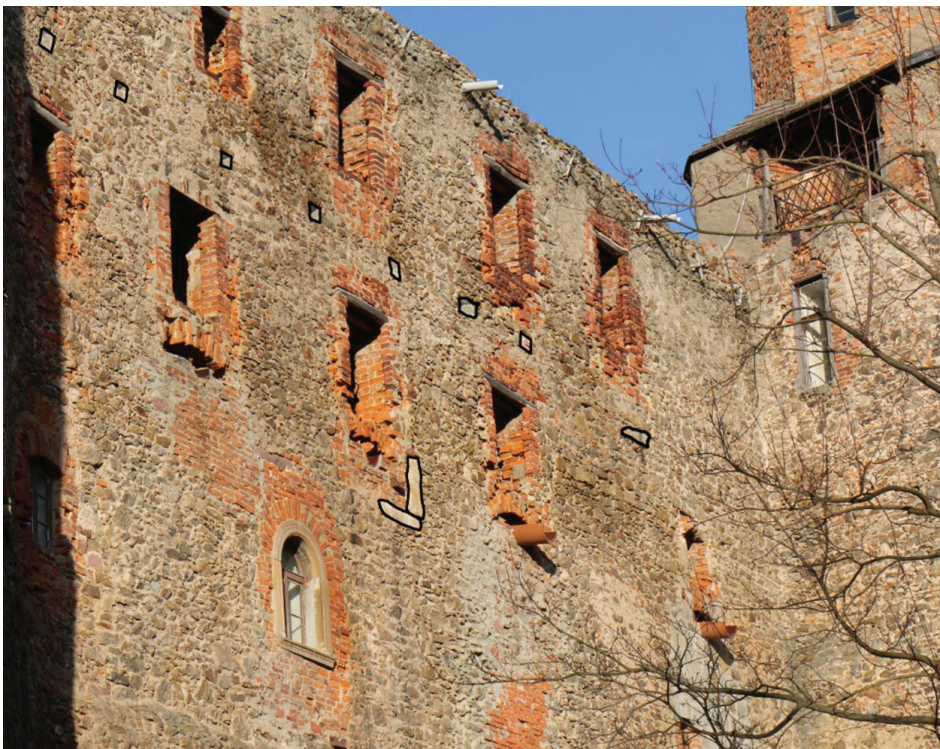
Fig. 8. Grodno Castle. View of the southern curtain of the perimeter wall. Nests of the cantilever beams of hoarding and relics of late gothic window stonework were outlined (photo by M. Chorowska)
