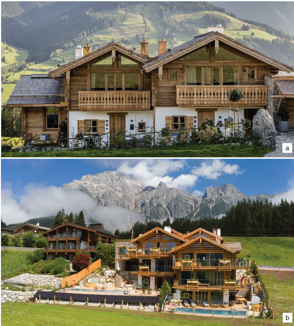
Fig. 10. Leogang, Senhoog hotel complex, design and construction management by W2 Manufaktur, Bmstr. A. Waltl, arch. B. Krynicka; façades: a) north, b) south (source: W2 Manufaktur)
