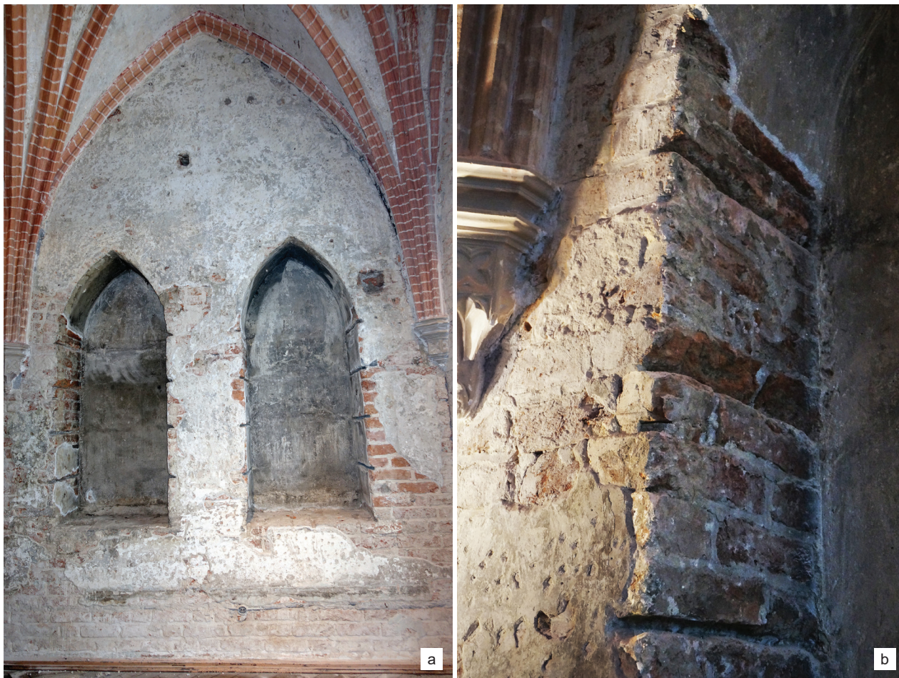
Fig. 5. The northern bay of the western wall with a pair of ogival recesses. Their side walls contain horizontally bevelled and right-angled cuts so that shelves could be fitted: a) general view, b) detail with cuts in the southern wall of the second recess from the north (photo by A. Piwek)
