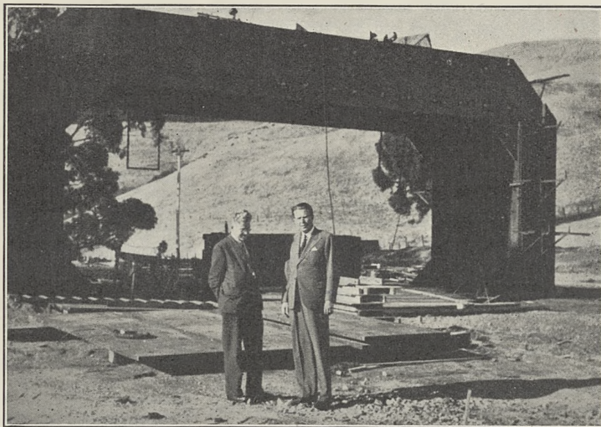
MAGNET OF THE 184-IN. CYCLOTRON UNDER CONSTRUCTION AT BERKELEY, CALIFORNIA.
