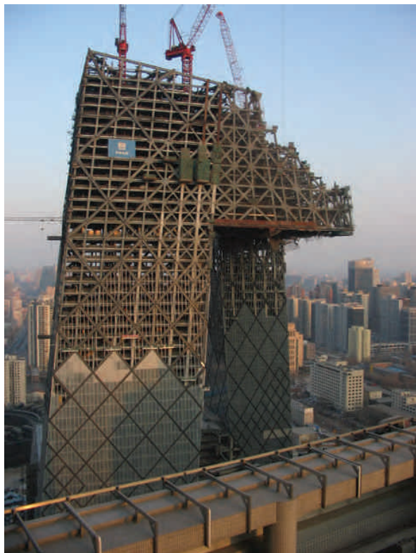
Fig. 7. Seat of CCTV in Beijing under construction (February 2008) designed by OMA. Futuristic structure is one of the 'icons' of modernized capital city of China (photo: J. Krajewska)
