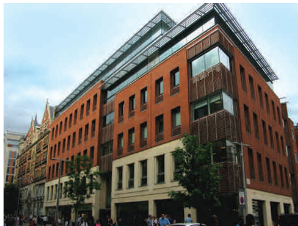
Fig. 6. Continuation of local tradition in modern architecture of London is exemplified by, inter alia, combining bricks in higher storeys with light service basement (stone, plaster) (photo: J. Krajewska)
