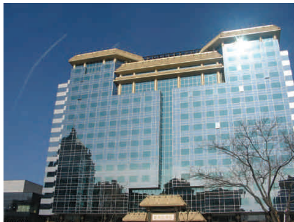
Fig. 3. Example of combining the modern architectural form with stylised detail, Beijing (photo: J. Krajewska)
