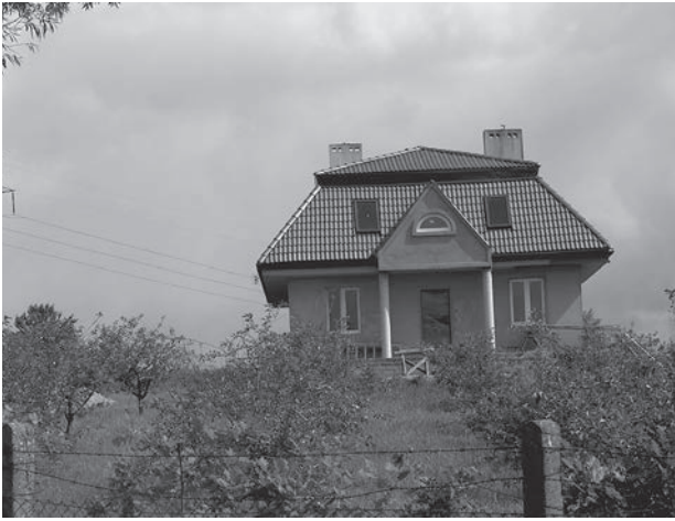
Fig. 9. One-family building in Siadło Dolne village near Szczecin – condition in 2008. Photo by author
