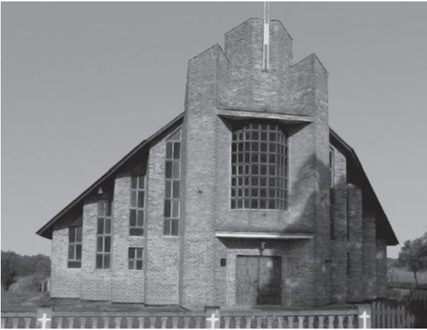
Fig. 5. Church in Chomętowo village, according to the design by Jerzy Koniński. Built in 1988–1996. Photo by author
