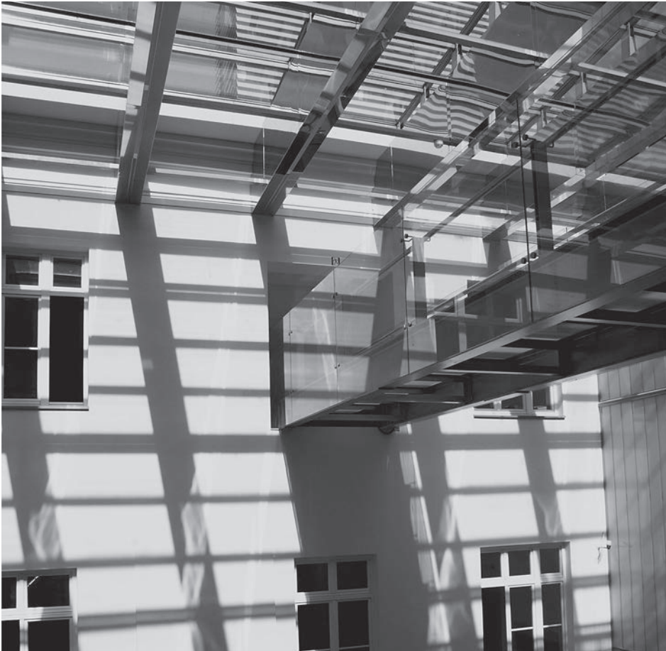
Fig. 1. Roofing the courtyard of Pod Kruki House. Photo by author
