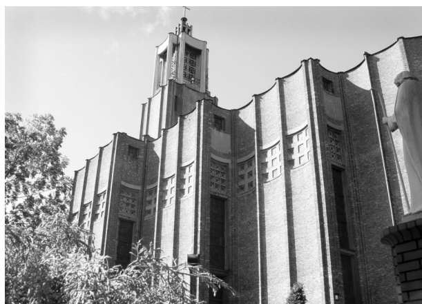
Fig. 14. St. Anthony's Church – fragment of side façade, existing state [2]
