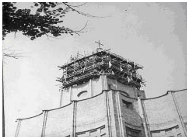
Fig. 6 Building of the reinforced concrete tower top [1]
