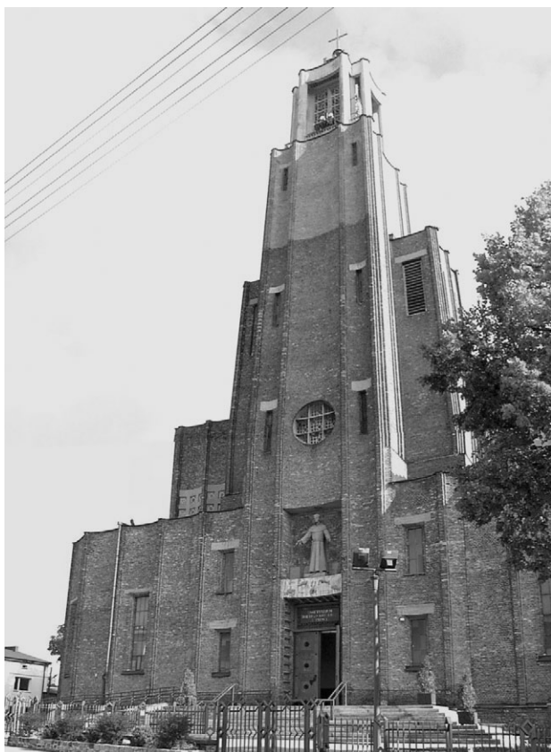
Fig. 12. St. Anthony's Church – front façade, existing state [2]
