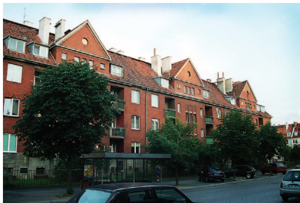
Fig. 5. Wrocław, the building of the J. Gotthelf Foundation, frontal elevation, photo 2005
