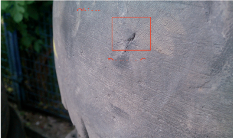
Fig. 11. Damage in object 16
