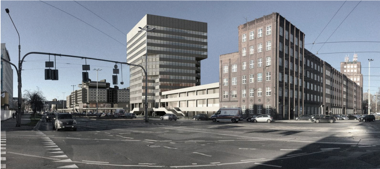
Fig. 6. Visualisation of the mixed-use centre at Dominikański Square, designed by J. Grabowska-Hawrylak, in cooperation with: K. Sęsiadek (1972–1976) – view from Traugutta Street, with the tower building that is part of the Main Post Office extension in the foreground, designed by J. Grabowska-Hawrylak, in cooperation with: J. Kaśnicki, K. Sęsiadek (1971) (model and visualisation by Ł. Wojciechowski)
