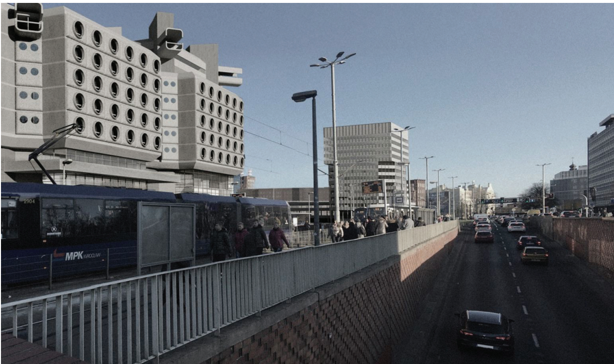
Fig. 7. Visualisation of the mixed-use centre at Dominikański Square, designed by J. Grabowska-Hawrylak, in cooperation with: K. Sęsiadek (1972–1976) – view from the side of Dominikański Square, with the tower building that is part of the Main Post Office extension in the background, designed by J. Grabowska-Hawrylak, in cooperation with: J. Kaśnicki, K. Sęsiadek (1971) (model and visualisation by Ł. Wojciechowski)
