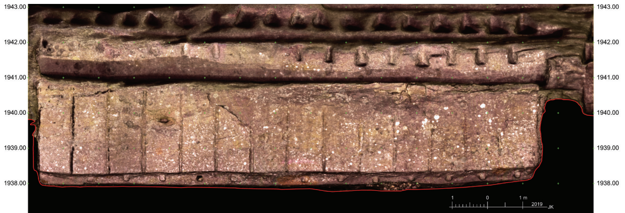
Fig. 38. The back wall of the room in the lowest part of sector S10
